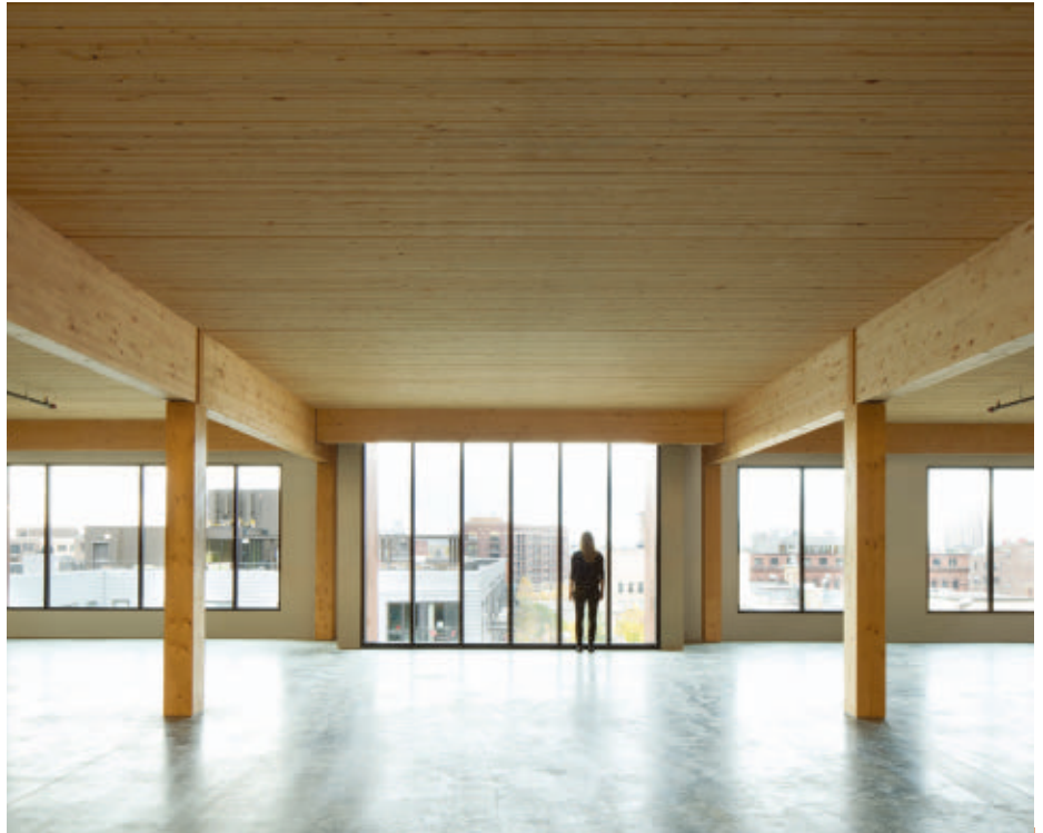
Exposed timber beams and ceilings at T3, a seven-story, 220,000-square foot office building in Minneapolis, were designed to attract creative tenants.
