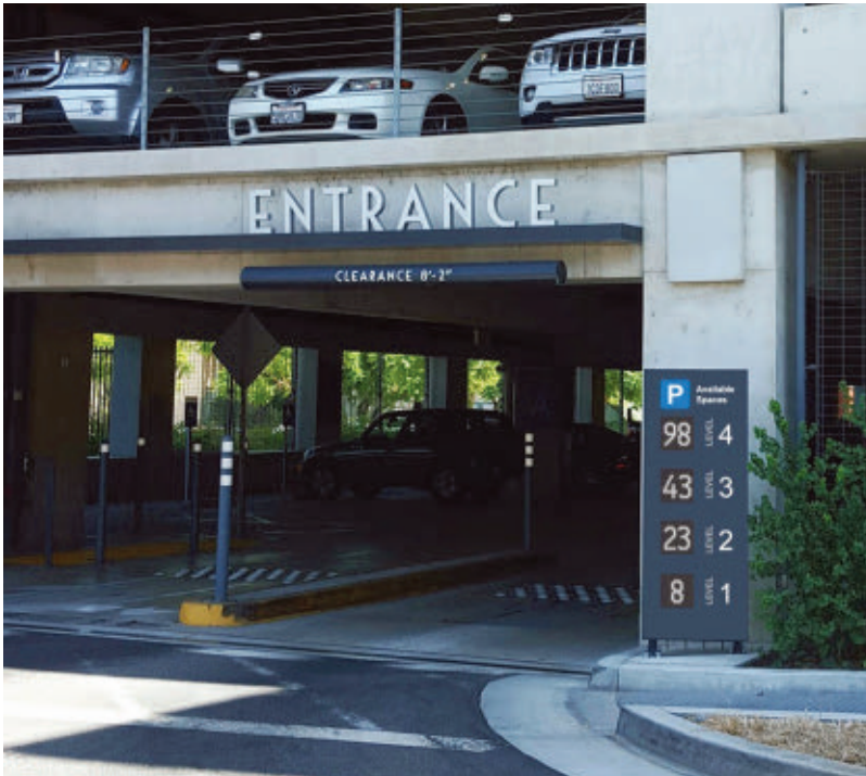
The parking guidance systems that measure occupancy also inform parkers where open spaces can be found within the parking facility.
