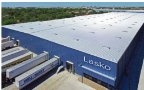
88 4x8 SKYPRO Polycarbonate Skylights GC: Sedalco City: Fort Worth, TX
