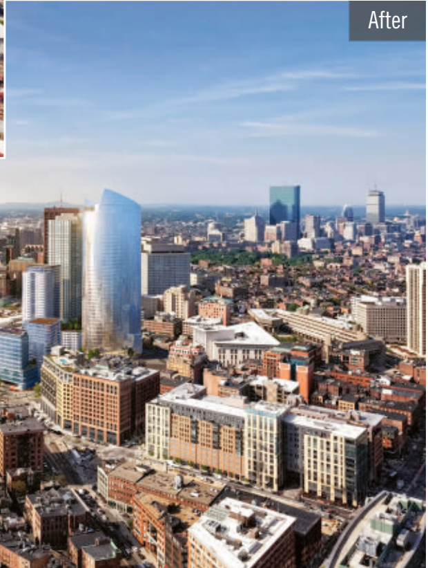
The site of the massive Government Center Garage (at lower right in “before” photograph) site is being redeveloped as the 4.8-acre, 2.9 million-square-foot mixed-use Bulfinch Crossing,
