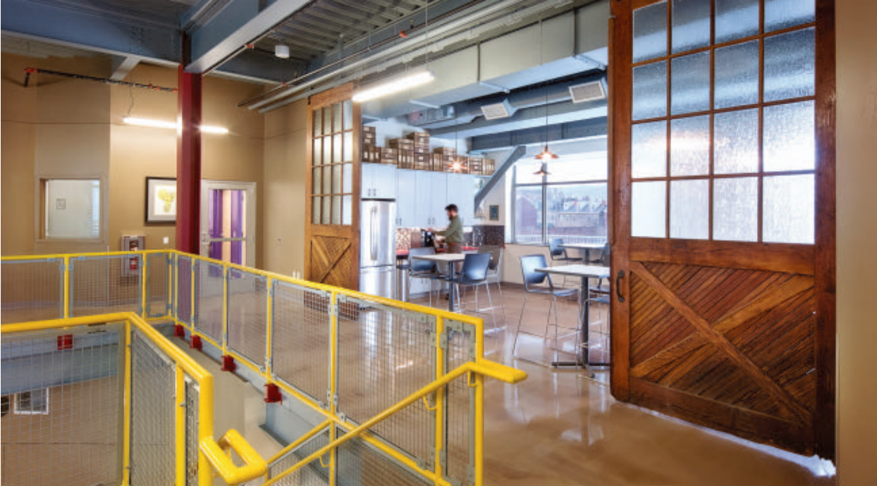
The structure's original wooden delivery doors have been repurposed as sliding doors to an employee break room.
