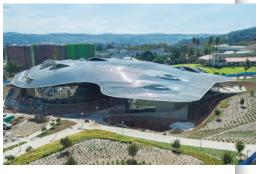
electrical devices, the roof collects, stores and distributes solar energy in the form of heat in the winter and rejects solar heat in the summer.
