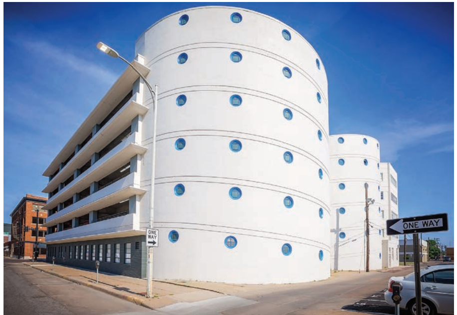
The Broadway Autopark, a historic parking garage in Wichita, Kansas, that was built in 1949, was converted into an apartment building with 44 one-bedroom units in 2018.
