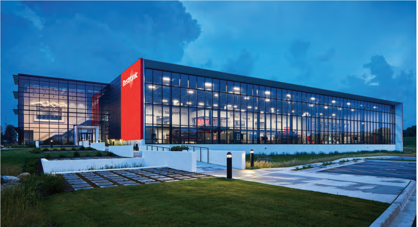
The Bystronic "Experience Center" in Hoffman Estates, Illinois, combines offices, warehouse space and manufacturing operations. It is the North American headquarters for the Swiss machinery manufacturer.
