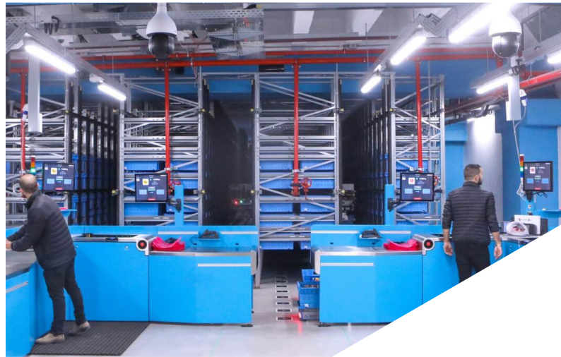
An underground Fabric storage and retrieval system in Tel Aviv. ■ Source: Fabric.
